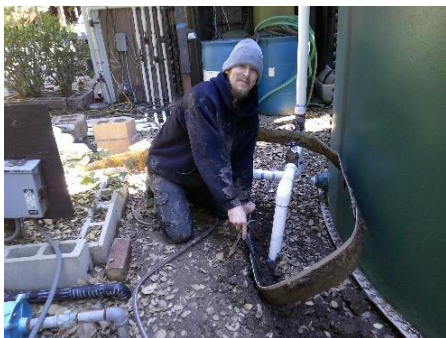
Luke from a local parish works on our ailing water tank.
