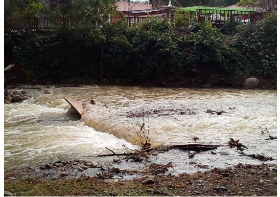
Our homemade footbridge, submerged and partially bent out of shape in the recent deluge.
