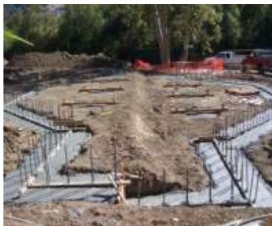
The building site as we go to press
